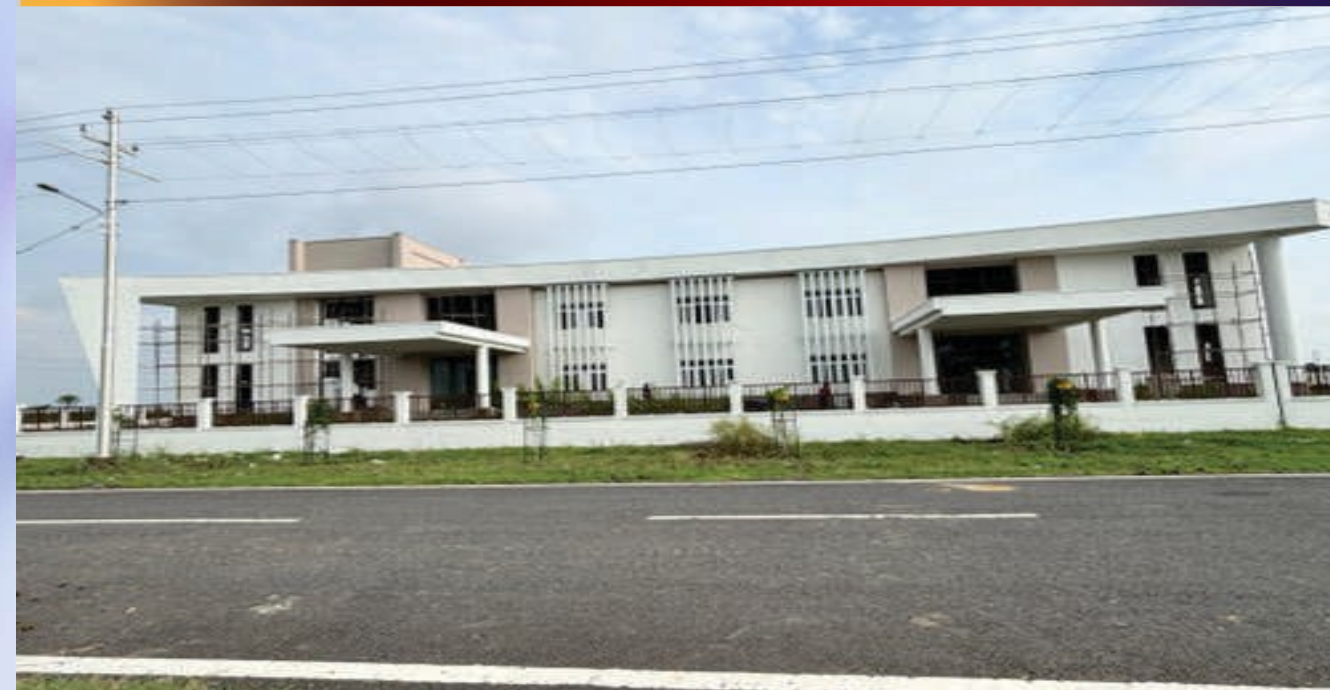
3-D view and actual view of CSF-5: Rapid Prototyping & Testing Lab
